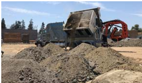
Dino unloading into stockpile on site.
